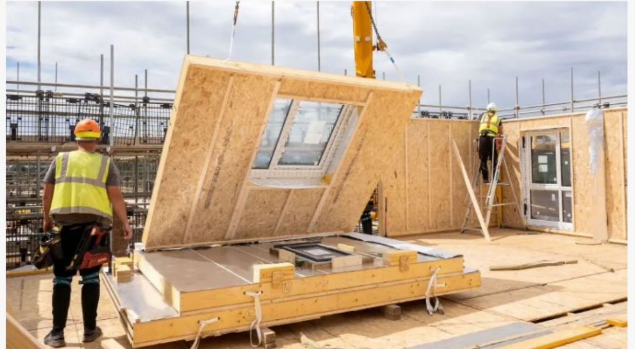
Sigma II panels, complete with pre-fitted windows, being installed onsite.; © Donaldson Timber Systems
